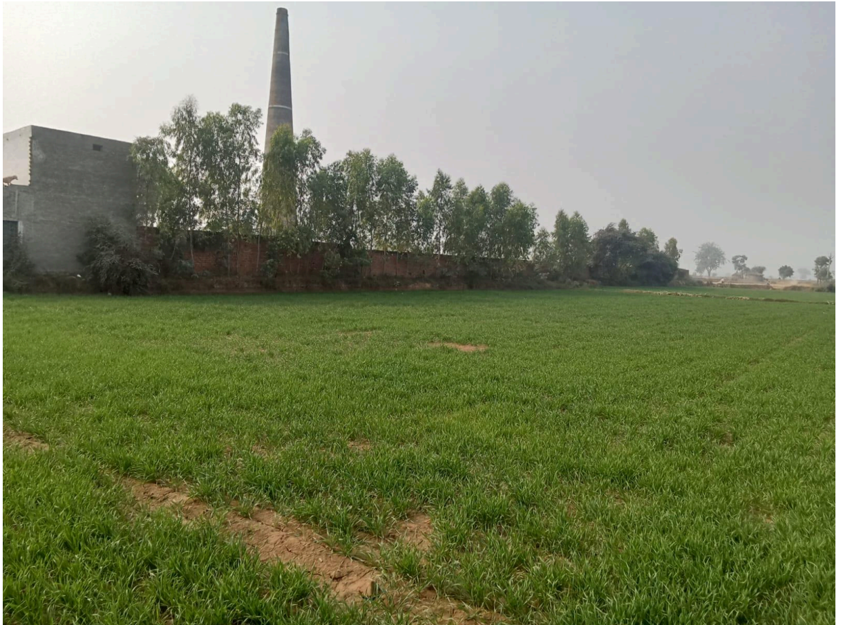
3-meter high boundary wall
